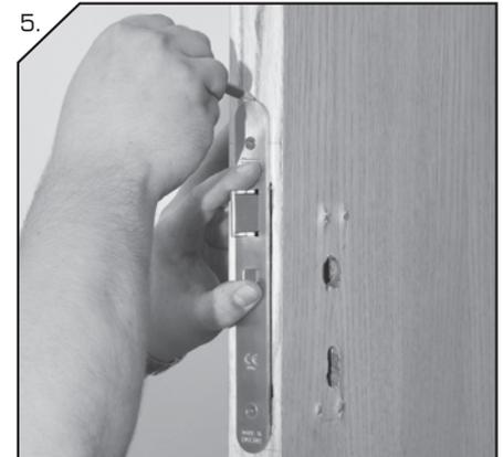
5. Taking care not to damage the cable, carefully insert the solenoid lockcase into the mortise and mark the faceplate position.
