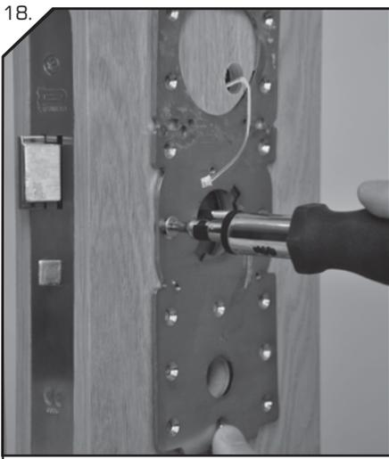
Re-fit the PASSPORT mounting plate push the 2 M5 Turn/Pull fixings through holes A1. Using the bolt through fixings, locate the screw ports on the back of the internal Turn/Pull and, taking care not to cross thread the screws, nip the screws up to hold the plate in position.
