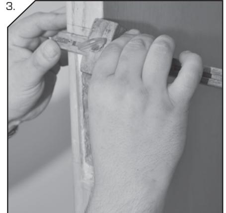
3. When the position of the lock is decided, mark out the mortise on the edge of the door as detailed more specifically at step 4.
