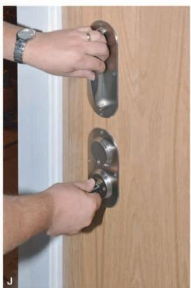
12. Offer the Doorstop on to the Frame Plate as shown at Fig I and re-lock by pushing the lever upright until it snap-locks into position. To check function and alignment use the Life-Line key to operate. Adjust accordingly ensuring that the door lock functions properly. Afterwards, remove the Doorstop and fully secure the Frame Plate to the door lining with the remaining 3/4" x 6 C/S woodscrews provided.
